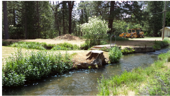
A sample of TUD's Ditch System
