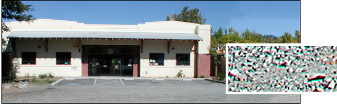
When the four paved spots at the Tuolumne Branch Library are full, patrons park in the unpaved Tuolumne Recreation Department lot.
