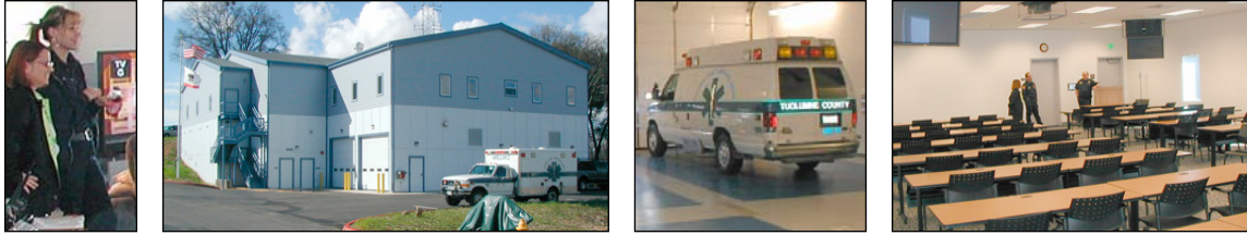
The recently completed 12,000 sq. ft. ambulance facility houses both the ambulance and TCFD administrative personnel and the 24-hour ambulance crew. The training room (far right) will be made available to county departments. It will serve as an emergency command center during large scale incidents.
